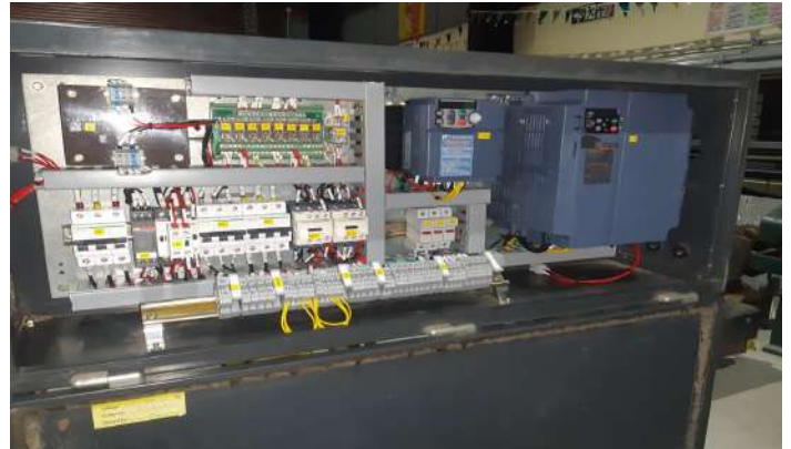
10 TON VFD PANEL FOR CRANE APPLICATION
